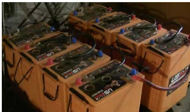
Figure 3- OGZEB battery storage system (two 48 V-battery arrays in parallel)
