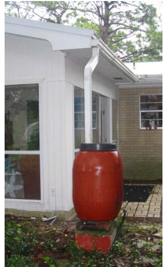
Figure 2. Rain barrels can supply a large portion of watering needs for many homeowners. Photo by Kathryn Ziewitz
