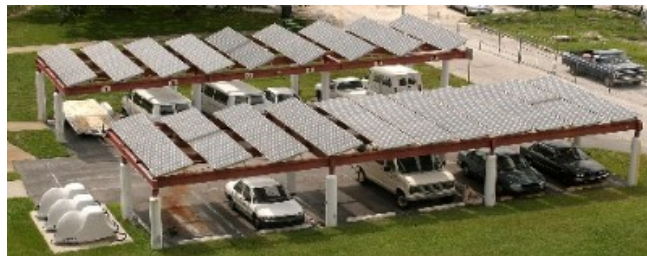
The original CERC PV array generated 20 kW of electricity. Presently, half of the system is being renovated with new PV modules to provide 10kW of electricity to be tied to the utility grid.
