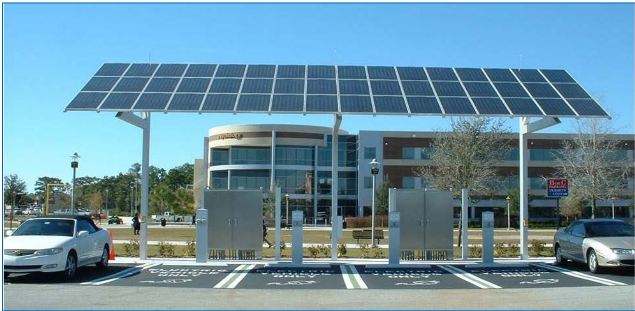
Solar Carport parking spaces on the UCF campus.
