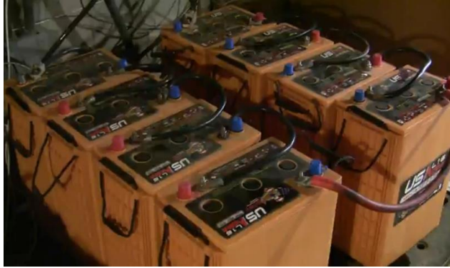
Figure 4- OGZEB battery storage system (two 48 V-battery arrays in parallel)
