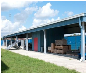
Figure 1: Ground Level Front View Completion
