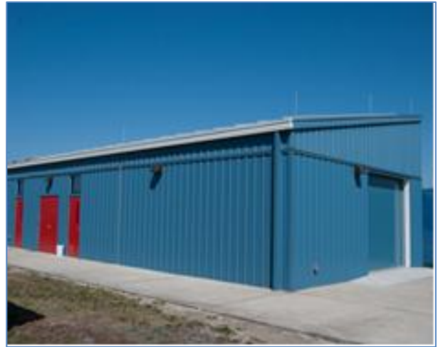
Figure 2: Exterior View after completion
