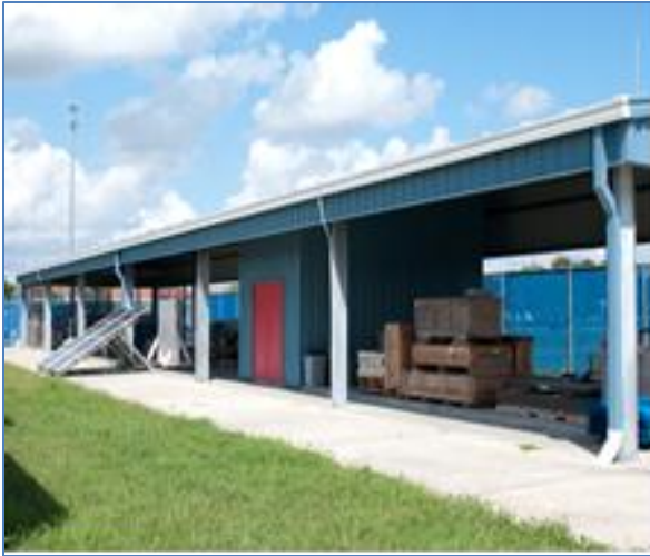
Figure 1: Ground Level Front View
