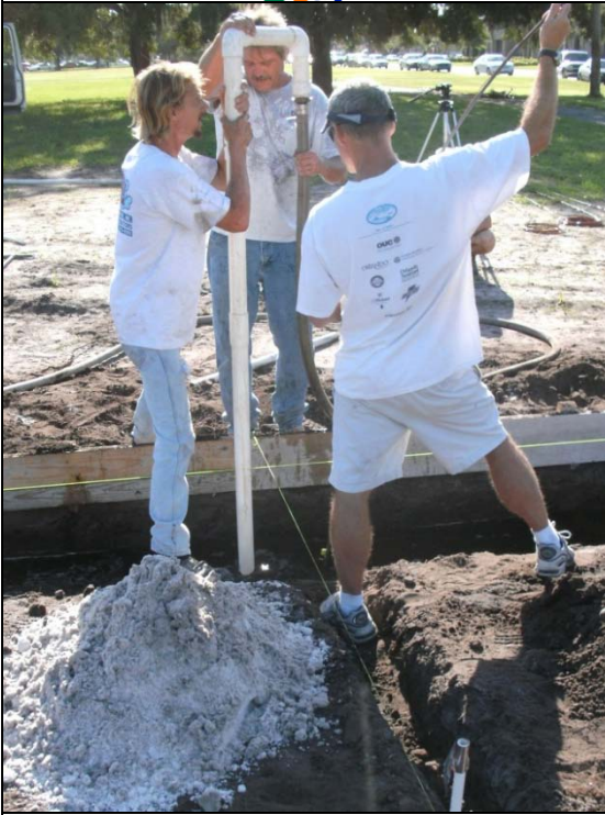
Figure 2. (above) Well is dug using water.
