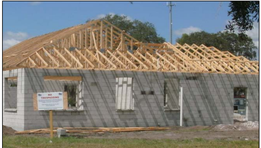
Figure 5. (below) Rafters were placed on the East house by hand.
