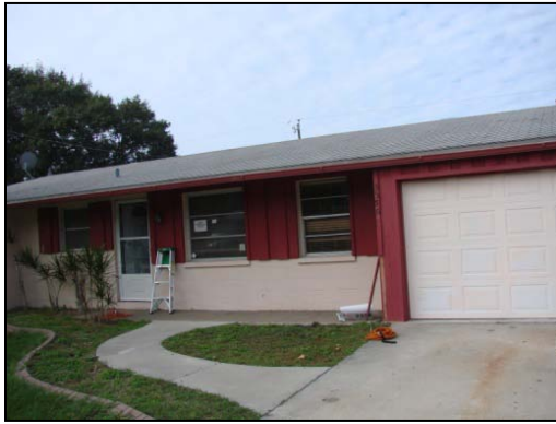
Sarasota County home before retrofit
