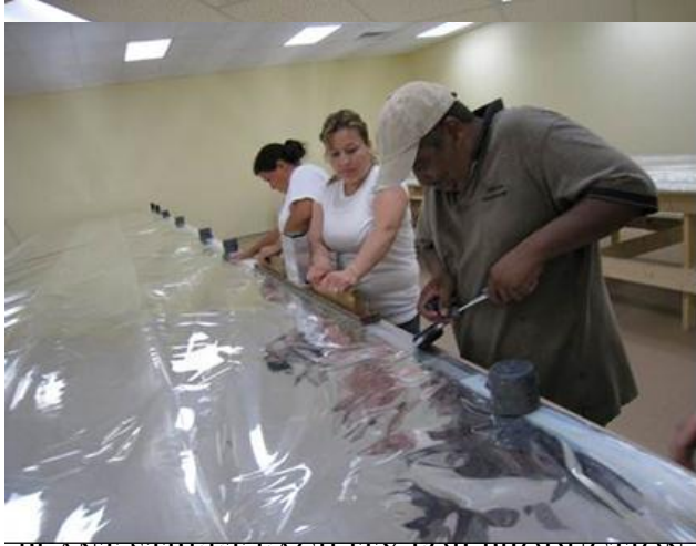
PLANT STREET FACILITY FOR PRODUCTION REHEATING THE GLUE TO BOND THE MEMBRANES TOGETHER
