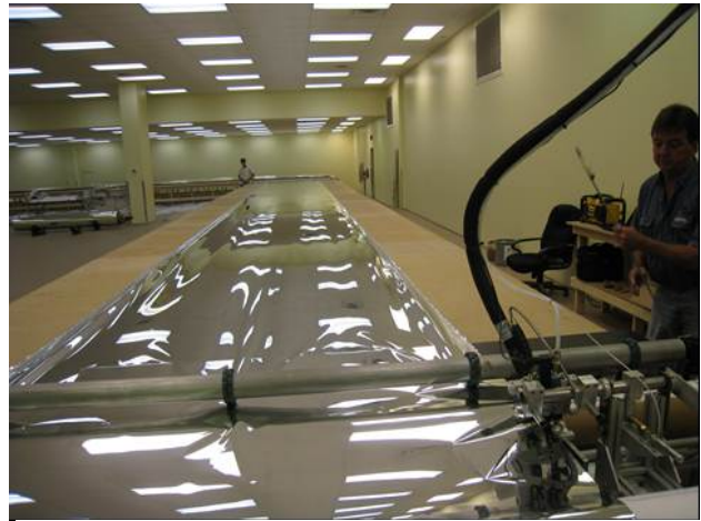
Applying Glue to Reflective Membrane
