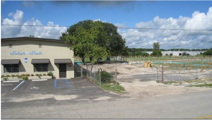
Street View of the Yulee St. Site From The East
