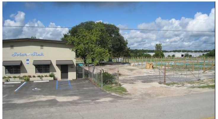
Street View of the Yulee St. Site from the East
