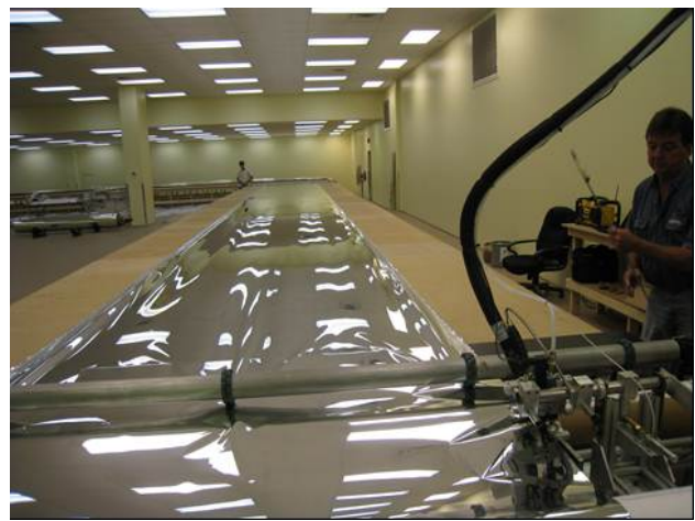
Glue machine applying glue to reflective membrane
