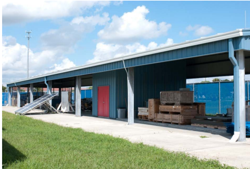
Figure 1: Ground level front view
