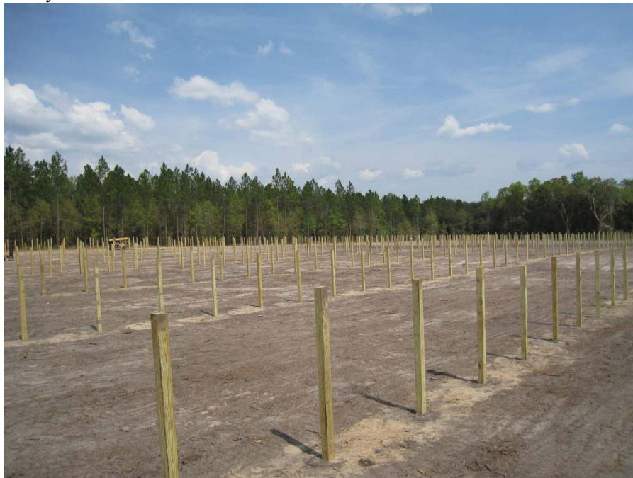
Posts installed at Site 3 (for 1800 balloons covering about 20 acres).
