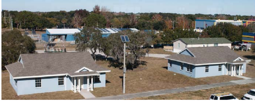
Completed flexible residential test structures on FSEC campus.
