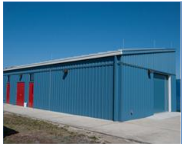
Figure 2: Exterior View after completion
