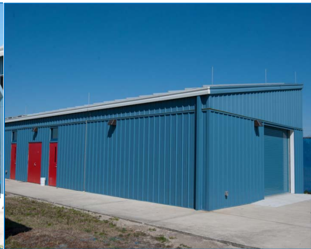
Figure 2: Exterior View After Completion
