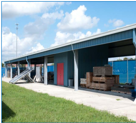
Figure 1: Ground Level Front View Completion
