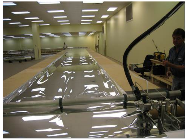
Glue machine applying glue to reflective membrane
