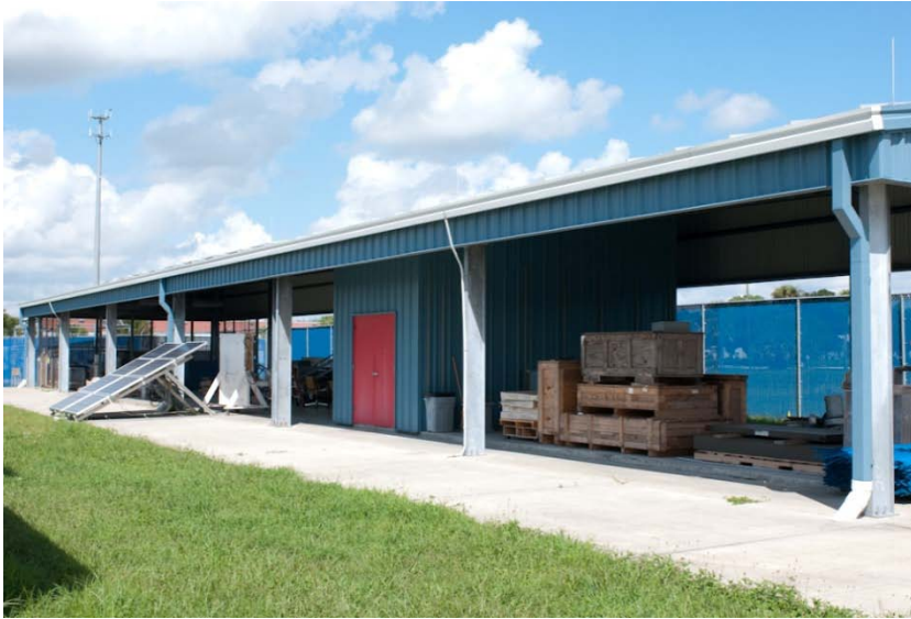
Figure 1: Ground level front view
