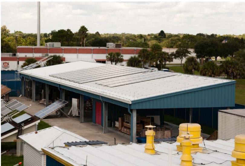
Figure 2: Roof view showing PV panels being tested.
