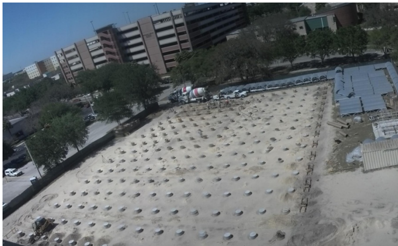
Fig.2. Solar Field for 50 kW e power generation
