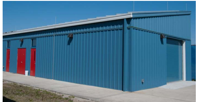
Figure 2: Exterior View After Completion
