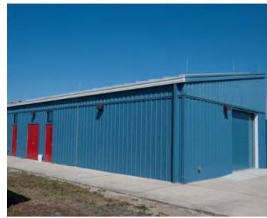
Figure 2: Exterior View After Completion
