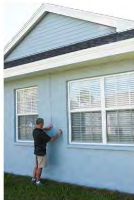
Senior Engineer, John Sherwin, installs wall surface thermocouple.
