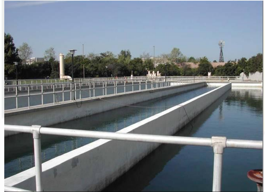
Traditional chlorination contact tank for water disinfection
